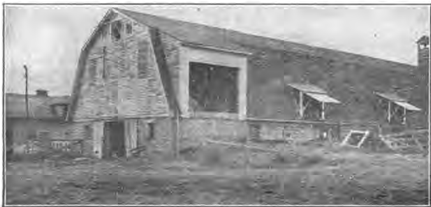
On G. C. Begent's farm in Tompkins County, N. Y., the chopped hay is blown into the mow and cured by a special ventilating system. The propeller fan is in the dormer window at the right, and there is a suction fan in the peak at either end of the barn.
