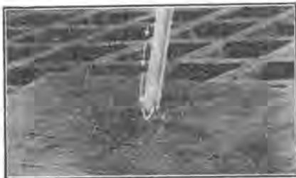
One method used by experienced welding operators to strike an arc. Electrode is bounced off the work and then returned to proper arc length. Arrow depicts direction of motion.
