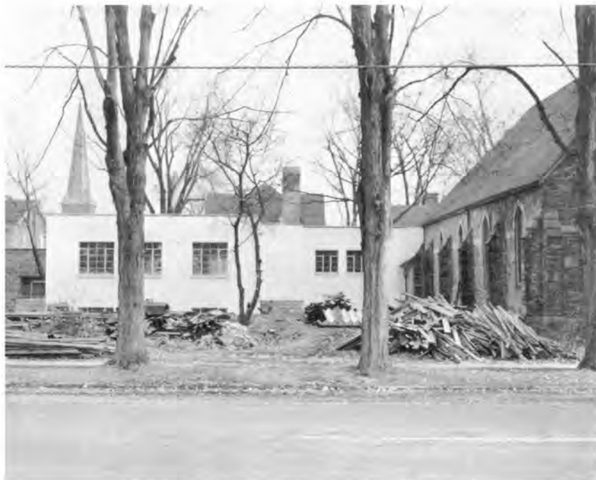
1949-1950 Addition to Christ Church nearing completion
