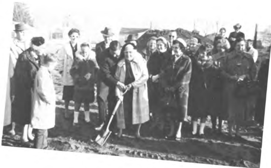
Groundbreaking for new Grange Hall — December 1962. Master Ann Ford and Town of Greece Supervisor Vincent Tofany turn over first shovel of dirt.
