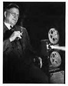
out of frame, you merely turn the framing knob and center the image without having part of the picture spill over the top or bottom of the screen. Once you've centered the projection "throw" on the screen you need not again retilt the projector to correct framing.
