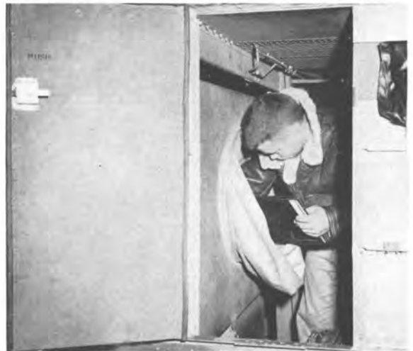
Exposed film is immediately processed by Corporal Donald Schewmaker, who is shown taking film through light trap. Thermos jugs prevent freezing of developing solutions
