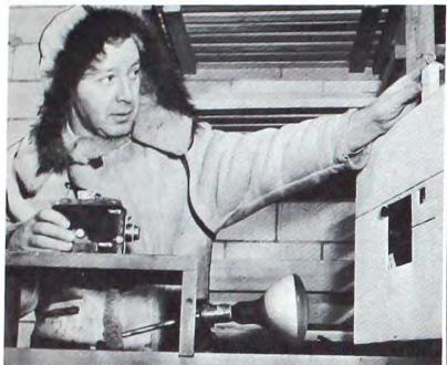
C-C-Cold - A lamb's-wool suit protects George Hastings from zero cold in the Low Temperature Room of the CW Testing Lab. This is the type of outfit worn by airplane pilots in high altitude flying. The cold room sometimes is held at 40 below, and a small cabinet can be maintained at 80 degrees below zero.
