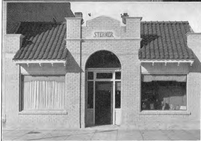
An example of what the advice of an architect and remodeling will do to a small studio. The old and new Sterner Studio, Moscow, Idaho.
