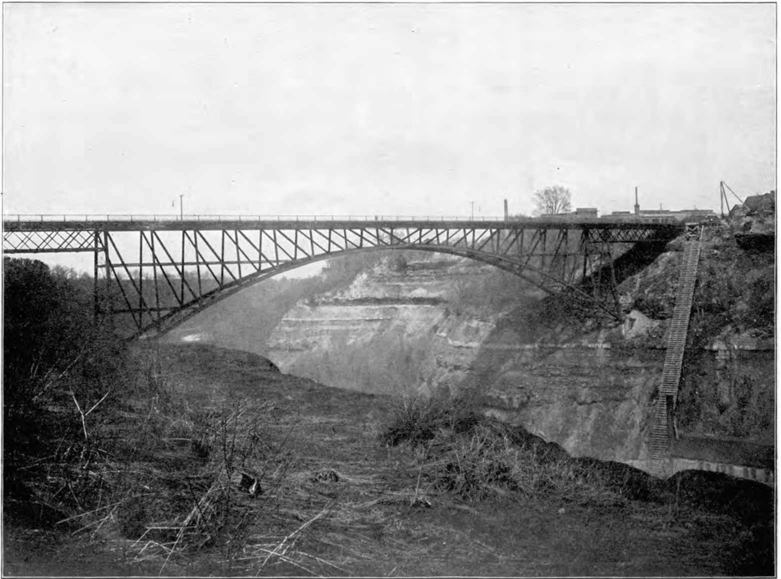
DRIVING PARK AVENUE BRIDGE
