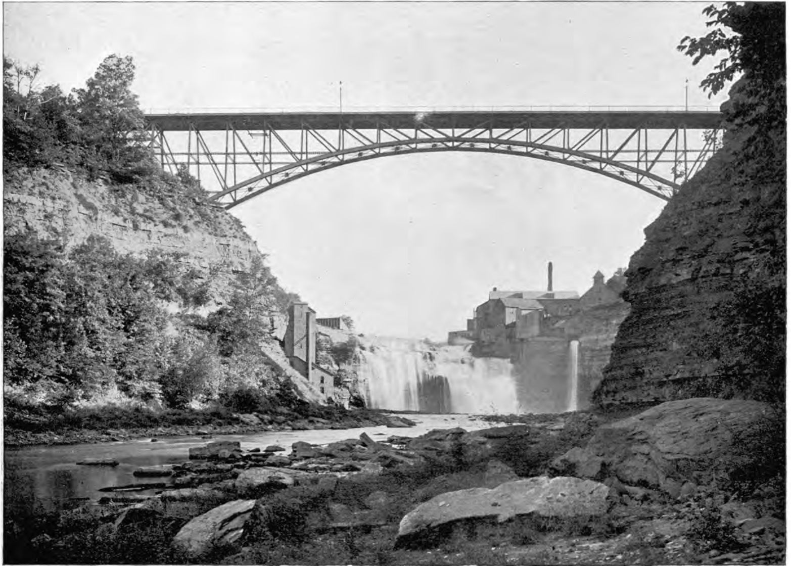
DRIVING PARK AVENUE BRIDGE AND LOWER FALLS OF THE GENESEE
